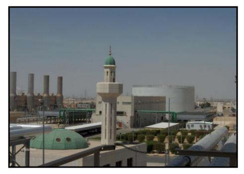
Chiller plant capacity31,000 tonsTES capacitynoneTotal project capital cost~\$75 millionNet power increase (6 h/d)~140 MWUnit capital cost~\$535/kW
