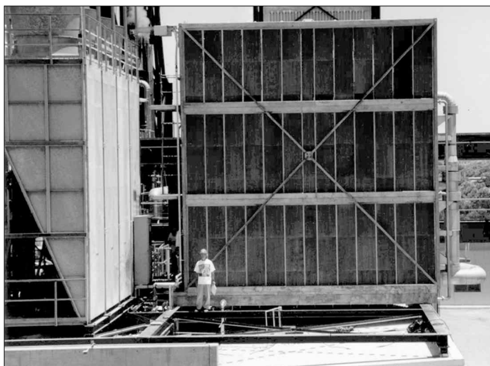
Figure 3. Retrofit of pre-cooler 2 x GT 8 in Chania/Crete.
