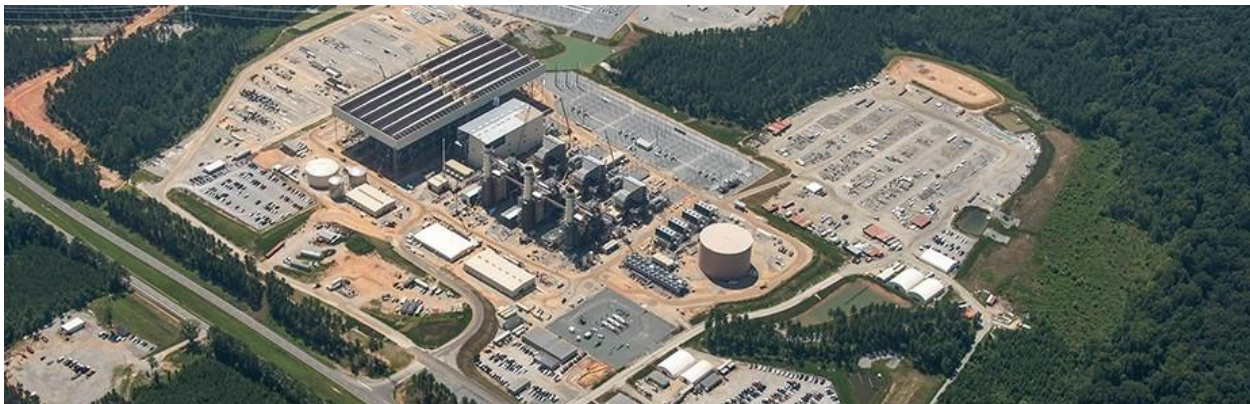
Photo 2 – Dominion’s Brunswick County, Virginia CTCC Plant with TES-TIC (Photo credit: Fluor)
