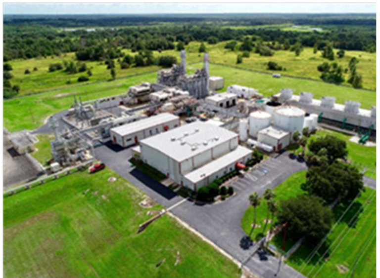
An aerial view of Orange Cogeneration Facility, Bartow, FL
