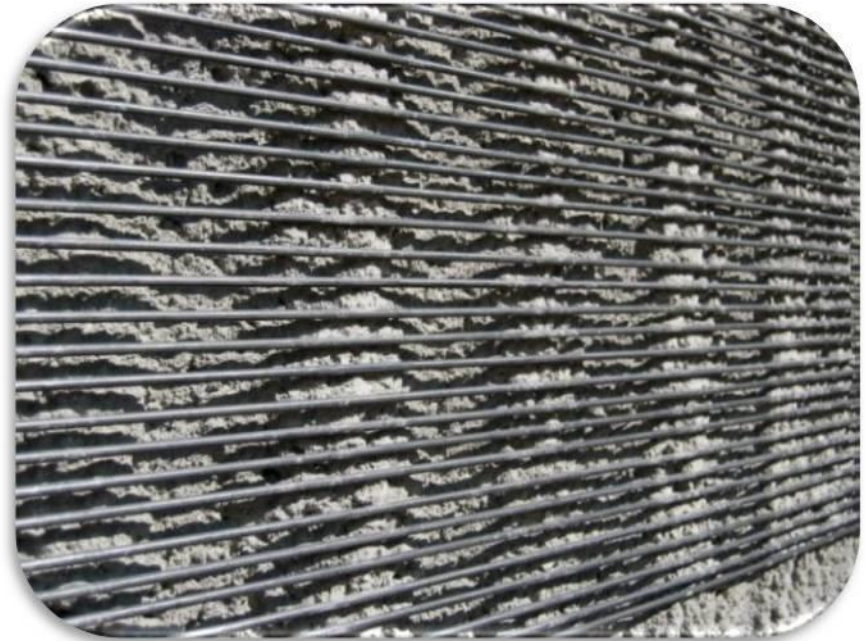
Pre-Stressing Calibrated Wire Spacing
